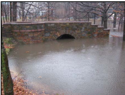
In December 2008, Riverway Island was inundated by flood waters.
